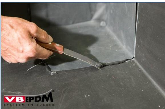
63. Remove emerging excess rubber adhesive.
