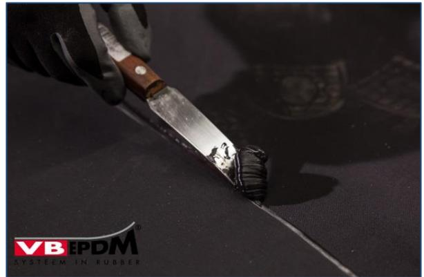
167. Removal of excessive sealant.
