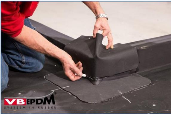
80. Marking upper part corner sealing sleeve.
