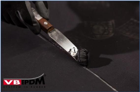
26. Remove emerging rubber sealant.
