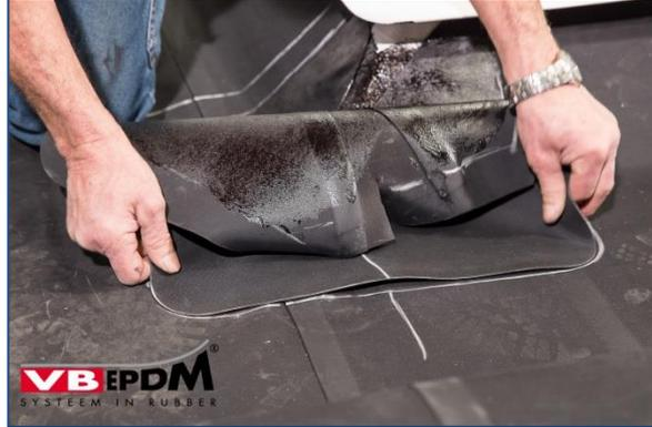
124. Placing prefab corner piece.
