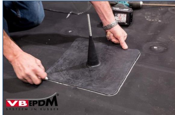
104. Positioning lightning conductor sealing sleeve.
