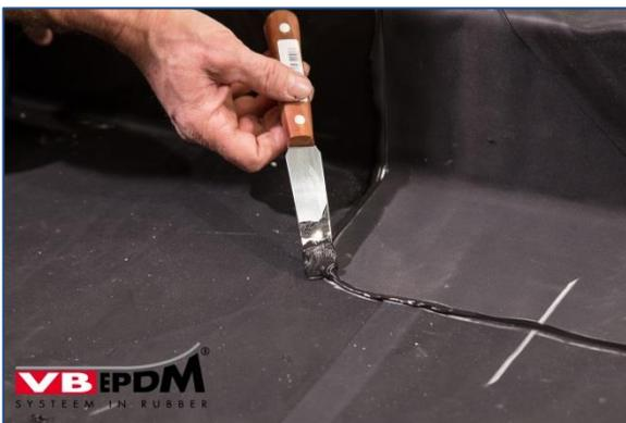
79. Remove excess sealant with blade.
