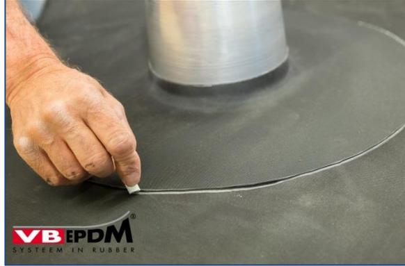
87. Marking sealing sleeve on membrane.
