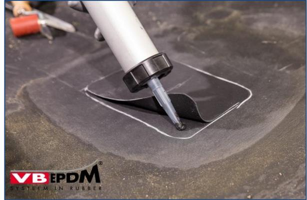
165. Sealing repair piece with VB-9510.
