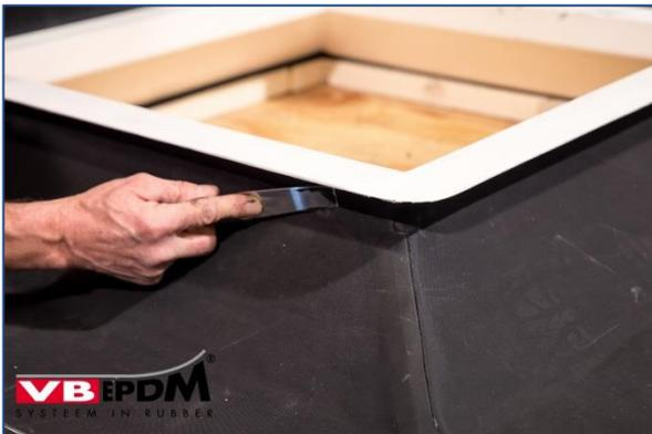
136. Folding shut sealing sleeve edge.
