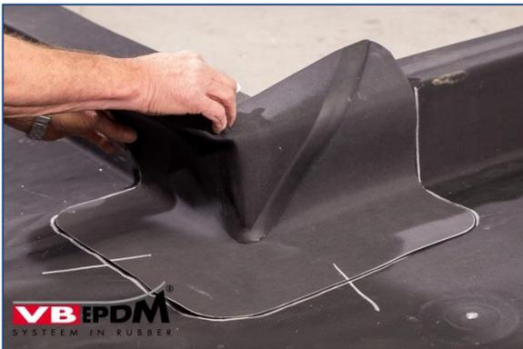
69. Positioning prefab outer corner piece.
