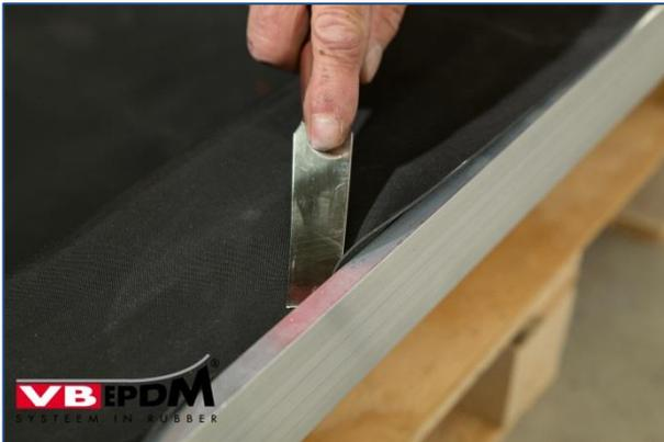
155. Sealing seal seam with blade.
