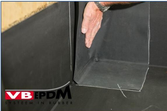
59. Rubbing sealing sleeve with flat hand.
