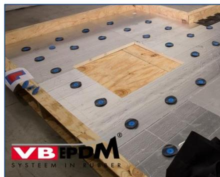
5. Thermofix® elements fastened.
