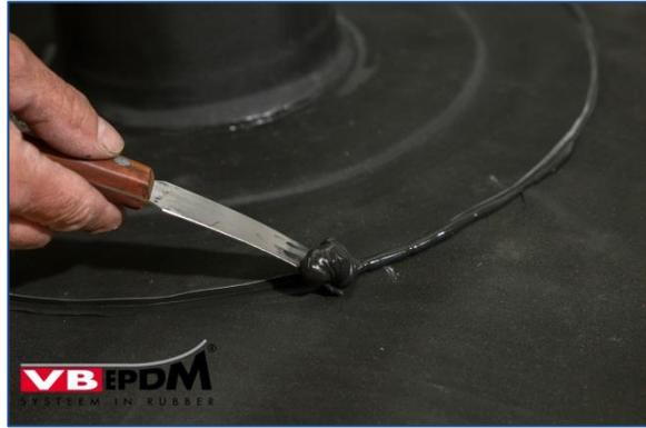
101. Remove excess sealant with blade.
