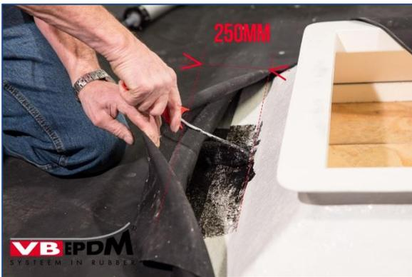
117. Gluing in dome upstand.
