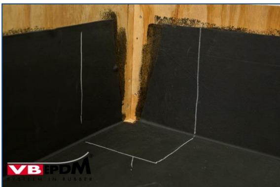
55. Sealing sleeve position marked on membrane.
