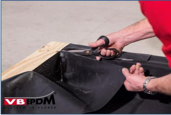
39. Cutting in inner corner with scissors.
