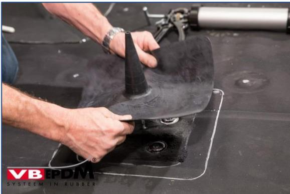
107. Placing lightning conductor sealing sleeve.
