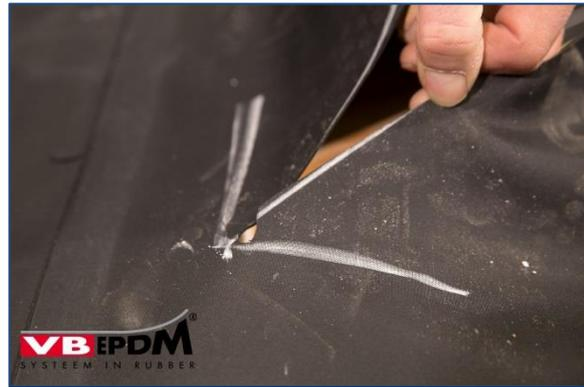
66. Cutting rounded off into membrane at outer corner.
