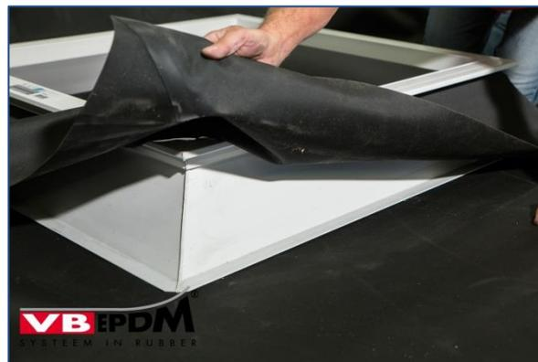
131. Positioning prefab sealing sleeve.
