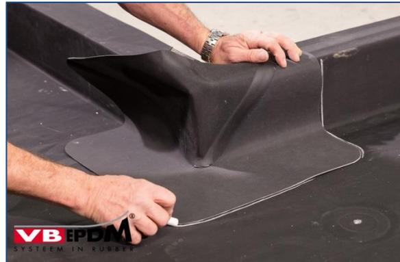
68. Marking prefab outer corner piece.
