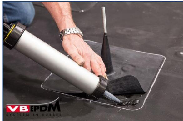
108. Sealing the sealing sleeve with VB-9510.
