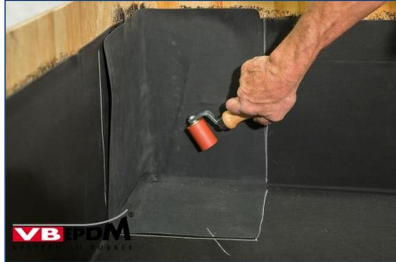
60. Rolling sealing sleeve with silicone roller.
